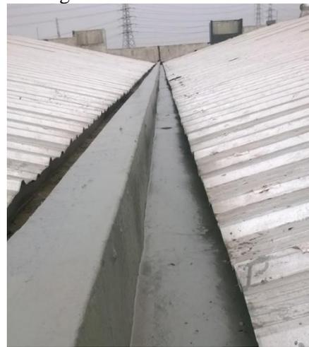
Gambar 6. Talang air Beton
